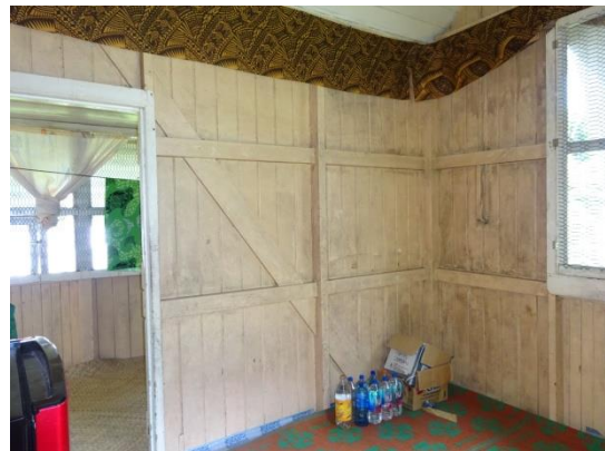
Fig.2-27 縦羽目板張内観
